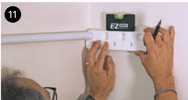
Level Tube and Tube Receiver on Right Wall. Mark four (4) screw holes. Collapse Tube (to left) as far as possible to allow for drilling of holes.
